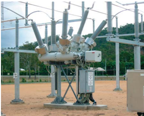
HGIS: Hybrid Gas Insulated Switchgear; Up to 550 kV HGIS Substation Solutions
